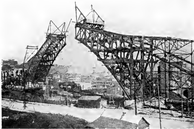
Fig. 3—Top chord Travellers lift steel from scows during erection of Cantilever.
